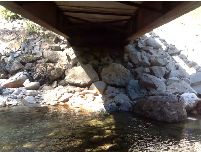
Left Bank Abutment when facing downstream
