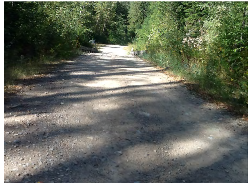
Right approach facing structure
