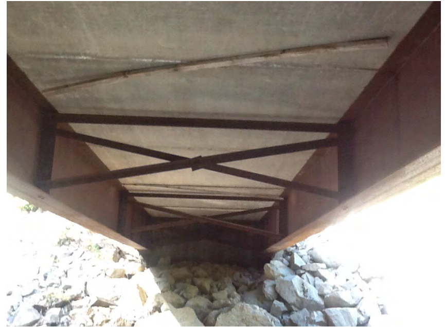
Underside of bridge
