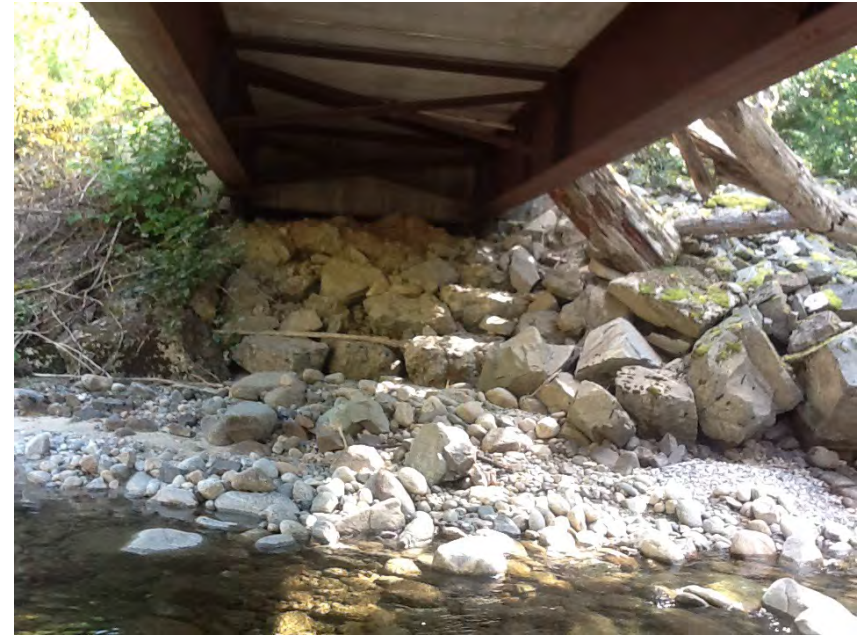
Right Bank Abutment when facing downstream
