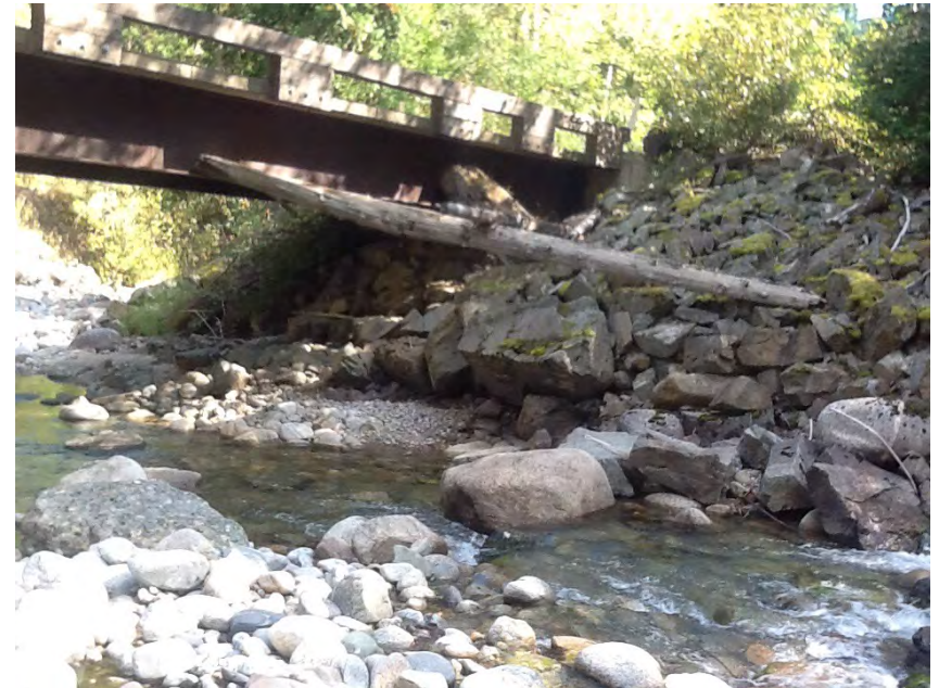
Right Bank Abutment when facing downstream
